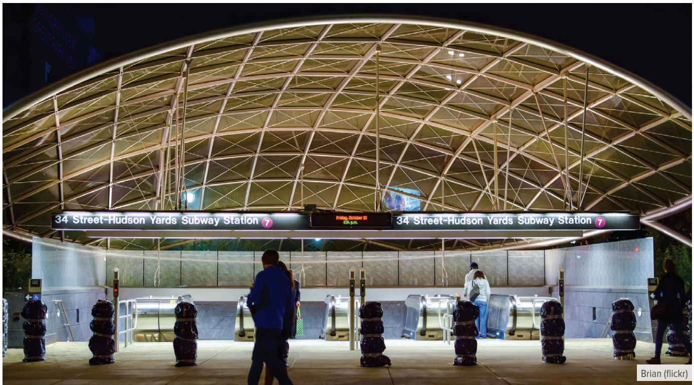
# 7 Line Hudson Yards Station Entrance
